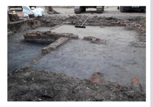
The picture shows the footings but an interesting Coal Chute was also discovered in one corner of the building along with a lower level floor which had an access from the kitchen. This can be seen on the left of the picture.
